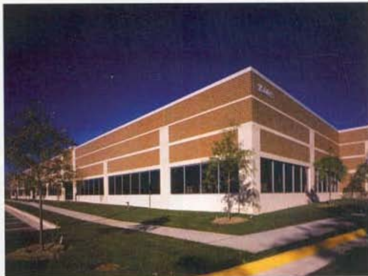
The Northridge at Westfield Office Park in Fairfax, Va., received a National Association of Industrial and Office Properties award. Photo courtesy of Smith-Midland Corp.
