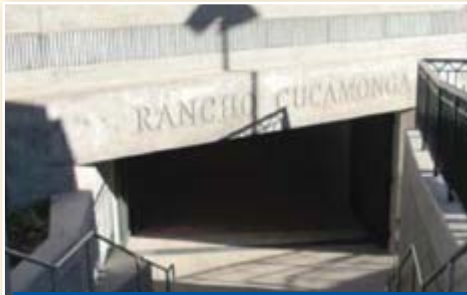
StructureCast Underground: 2 nd Place Pedestrian Undercrossing Rancho Cucamonga, CA
